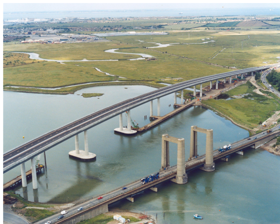
Photograph supplied by Carillion
