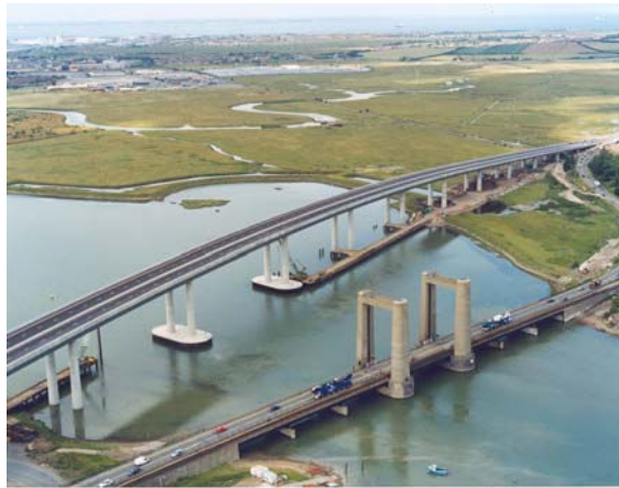
Photograph supplied by Carillion
